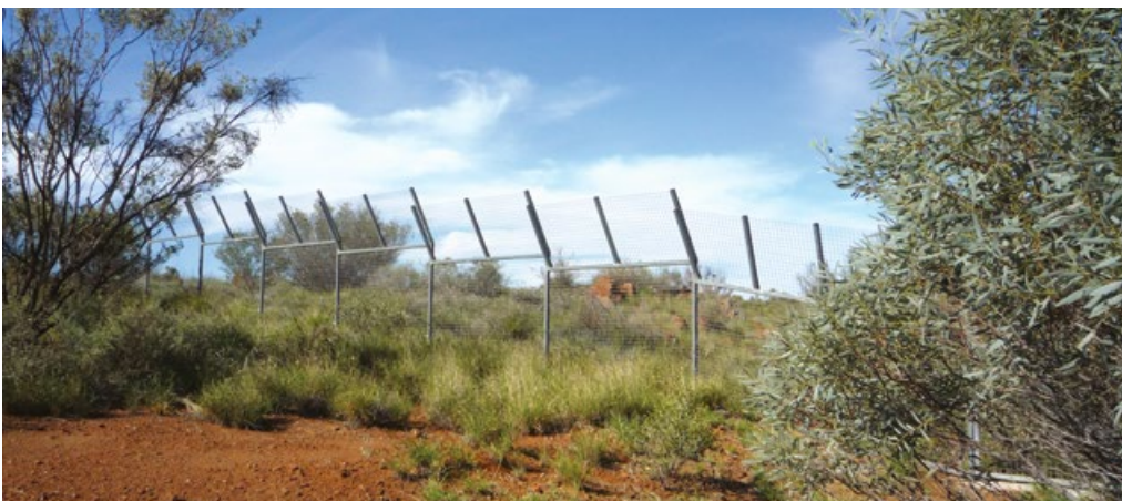
Perimeter fence at TPN
