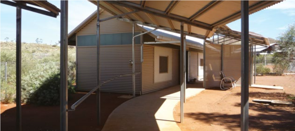
Sheltered path to bedroom unit at TPN
